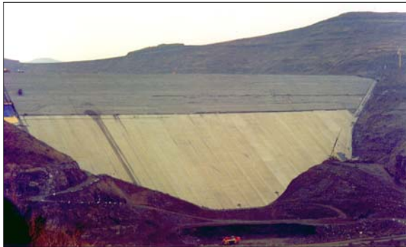
The Mohale dam during construction.
