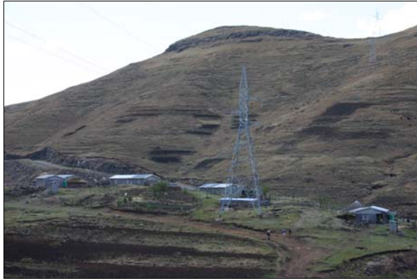
A pylon in the village but no power in the houses: the resettled village Ha Tsiu above Mohale Dam.
